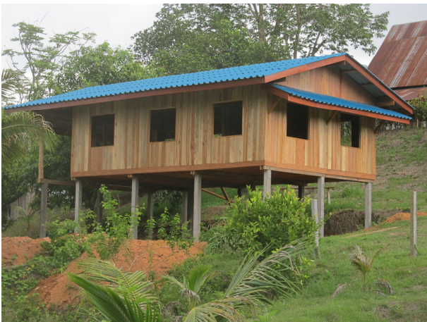
Staff house near completion (view from back side)
